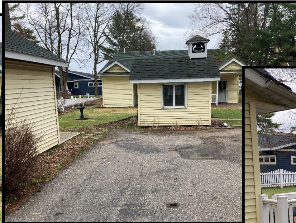
Storage Shed / Rear of Garage
